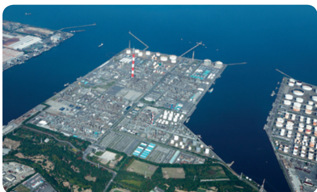
Oita Petrochemical Complex
